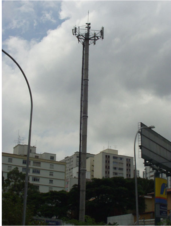
Fig. 1 Typical pre-cast RC telecommunication tower
